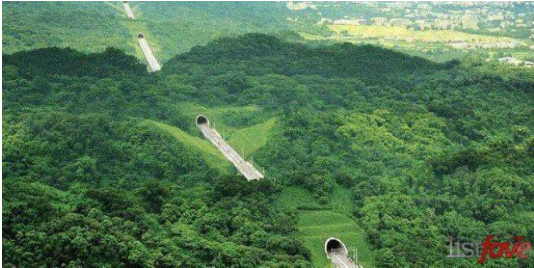
Hsueshan tunnel – Taipei, also known as "snow mountain tunnel"
