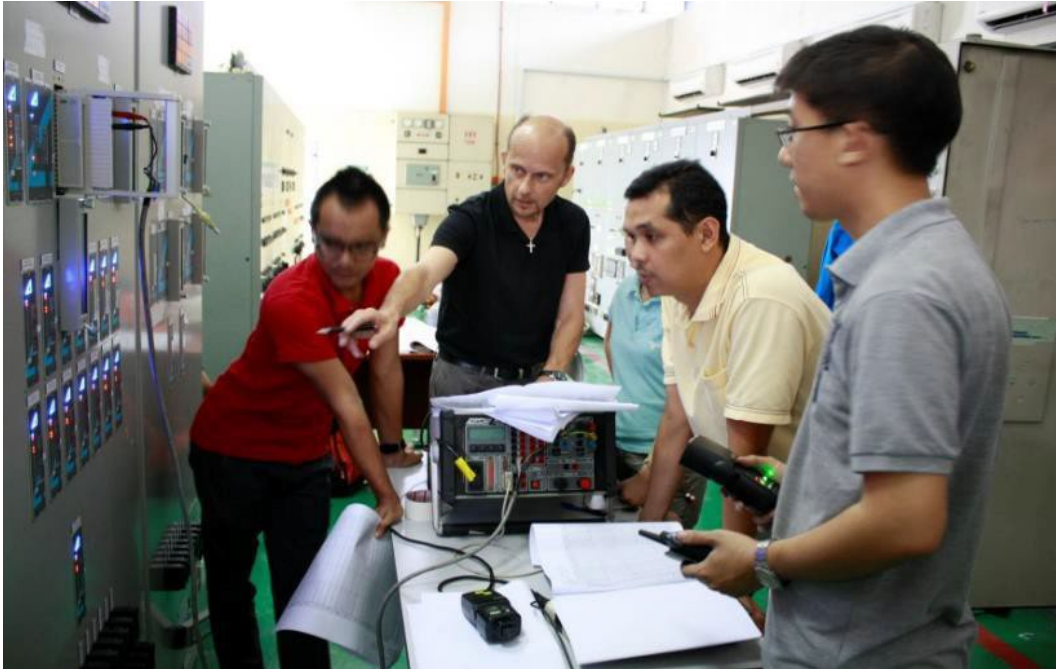
TNB arc protection approval test in 2013.
